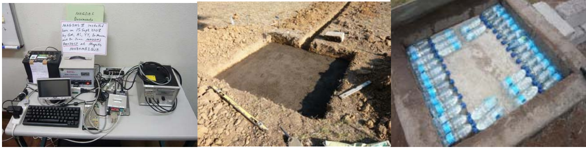
Fig. 6. Installation examples of MAGDAS-II (work by Africa B Team) (Left: Data Logging system at Maputo in Mozambique; Center: Cement base for sensor house at Lusaka in Zambia; Right: Water bottles for thermal stabilization at Maputo.)
