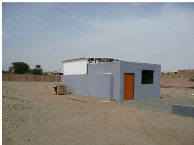
Fig. 2. New sliding roof for FMT in Ica, Peru.
